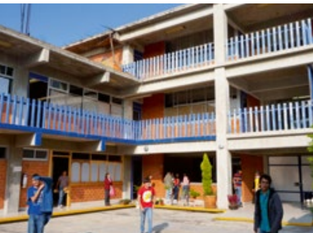
The courtyard from the new school building
